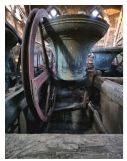
Wheels and fittings, in a poor and worn out state
